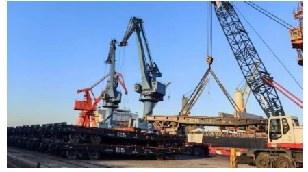
Malaysia East Coast Rail Link Project
